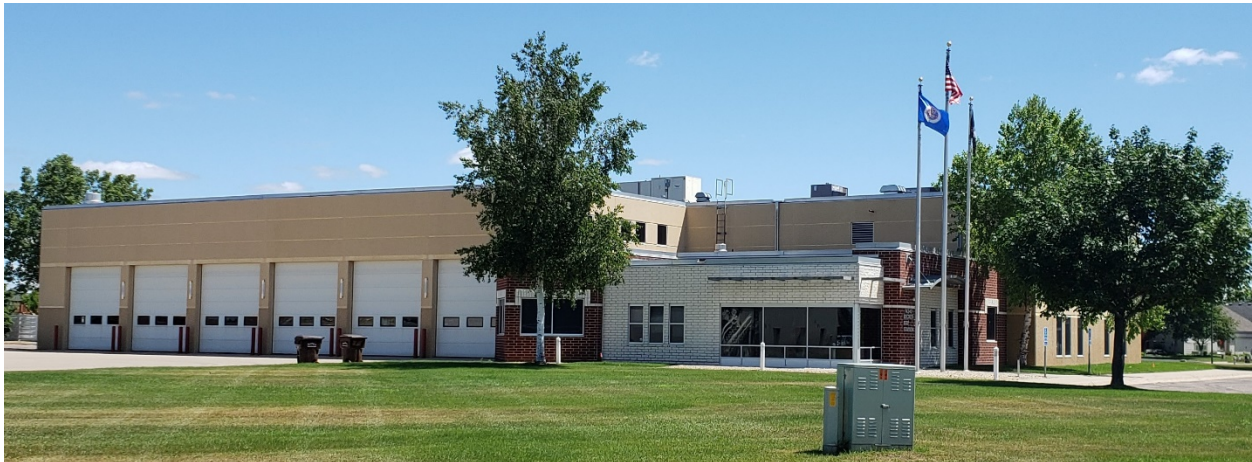
Current Fire Hall, June 2021
